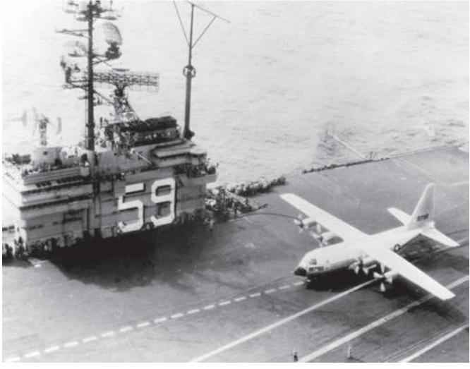
Engineers at the Naval Air Rework Facility in Norfolk, Virginia, figured out how to get the Hercules off the ship if, for some reason, it got stranded aboard the ship during the trials. The most practical solution would be to use I-beams and a large crane. "If we had broken down at sea, the deck hands would have lifted the plane up with the deck crane and tossed it overboard," crewman Ed Brennan mused
