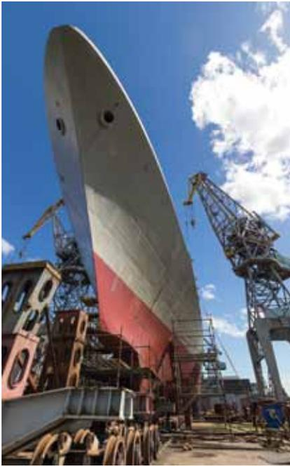
*Under the bow of the fourth 11356R/M frigate under construction at Yantar*
